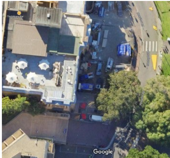
Figure 9: Waste bin location (2 red squares) – Loading dock off Hospital Road
